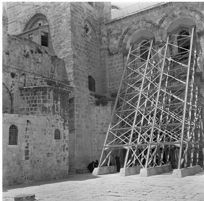
Image: Scaffolding supporting the Church of the Holy Sepulcher. 1950s, Jordanian Mandate of Jerusalem. Taken by Yousif Shamiyeh. All rights reserved.
